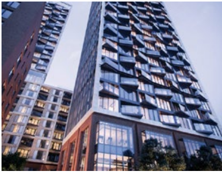
Portal West , London, UK
